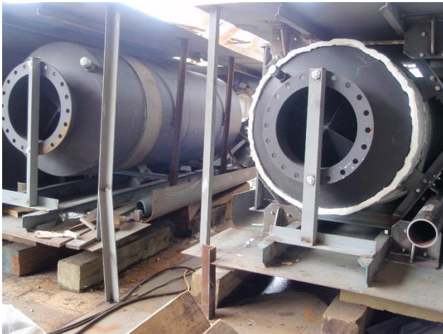
Silencer installation in exhaust stacks.
