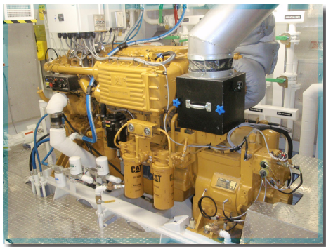
Twin 600-hp Cat engines power each of the new towboats.
