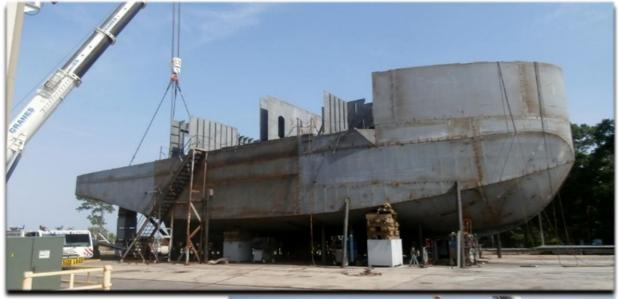
Patti Marine has completed the erection of the Moran 121' ATB hull modules with the stern installation this week. Deep South's 600 Ton Hydraulic Crane flipped and set the 207,000 lb. unit which completed the 3 month long hull erection process. Both main engines (6,000 horsepower EMD's) are already installed in the engine room. Our "Patti Built" crews have again proved their worth in speed and high quality workmanship!
