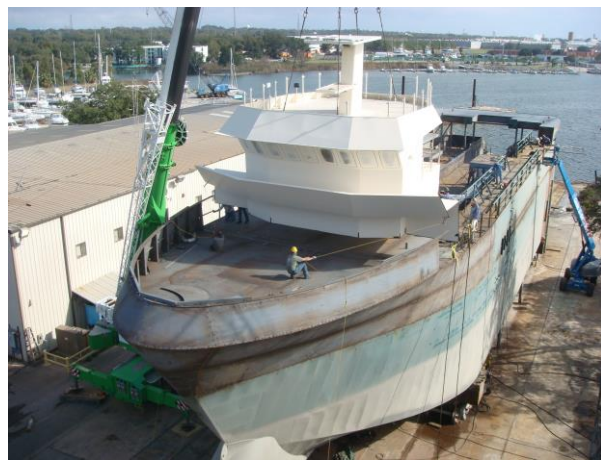
~ New Pilot House Installation ~
