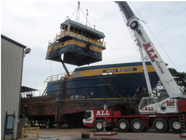
~ Old Pilot House Removal ~
